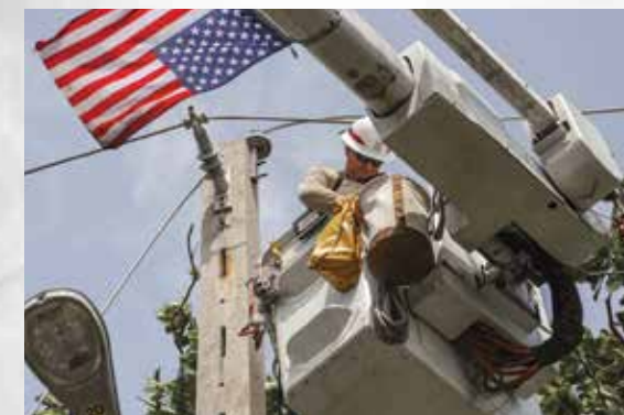
Above: U.S. Army Reserve Sgt. Eric Elder, a power distribution specialist assigned to Delta Company, 249th Engineering Battalion, U.S. Army Corps of Engineers, fixes downed power lines caused by Hurricane Maria to help restore power in the Rio Grande, Puerto Rico area, October 25, 2017. (Photo by Spc. Anthony Martinez)
